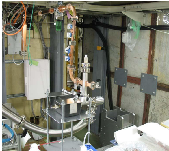
Figure 7: New concrete vault for test.
